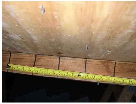
MEASUREMENT ROOF TO DECK ATTACHMENT
