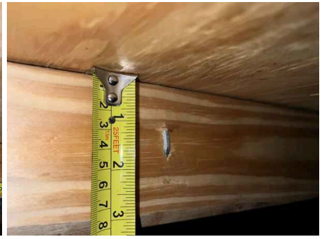
8D NAIL ROOF TO DECK ATTACHMENT
