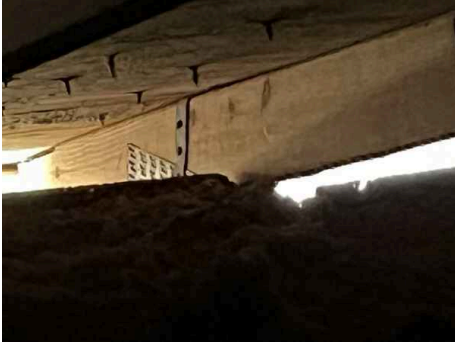
SINGLE WRAP ROOF TO WALL ATTACHMENT
